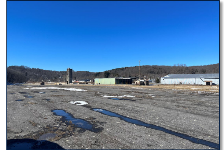
Existing Buildings and Silo
